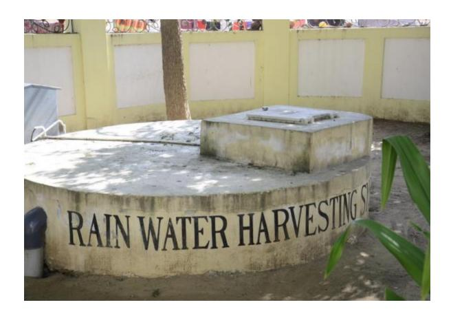
9. Brick work Tank behind residential block 234 (Capacity 15,000 Litres): It receives the rain water from the terrace of housing Blocks no. 233,234 & 500. The collected water is used to maintain green area to maintain park behind these housing blocks.
