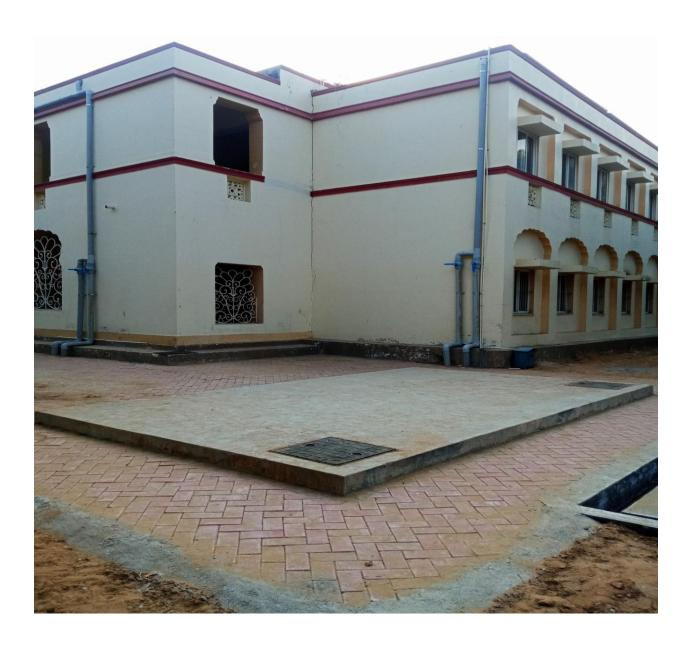
7. RCC Tank in Krishna Bhawan Hostel Premise (Capacity 50,000 Litres): It receive the water from some portion of Bhawan that is sieved through a Copper reinforced sieve slab making it drinkable that is sent back to the overhead storage tank that supply it in Water cooler and Toilet.
